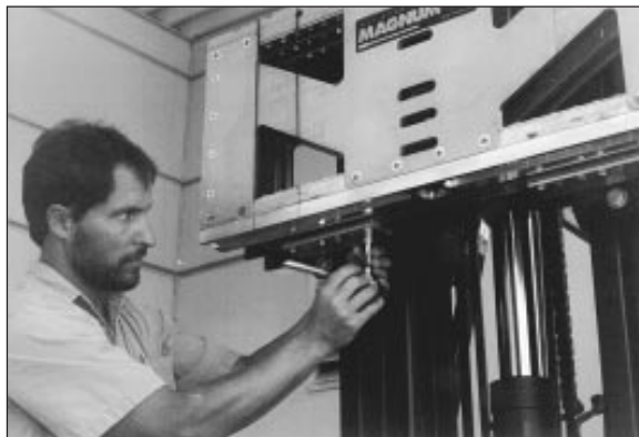
Figure 4: Attaching the safety plates.
