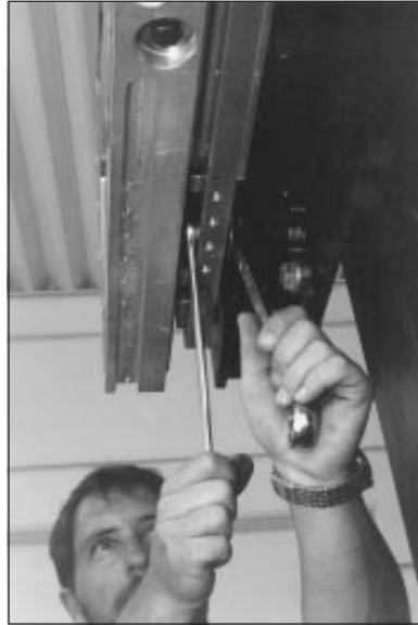
Figure 3b: Adjusting the jam nuts.
