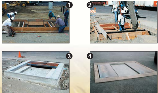
Typical in ground installation
